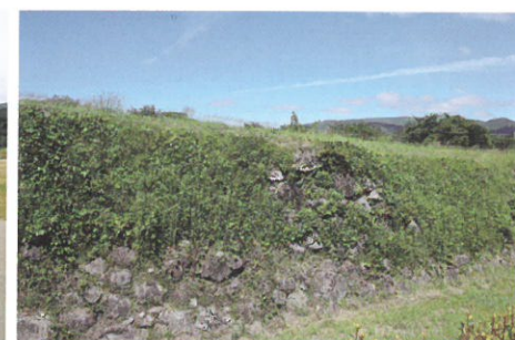
④本丸南側堀の石垣
